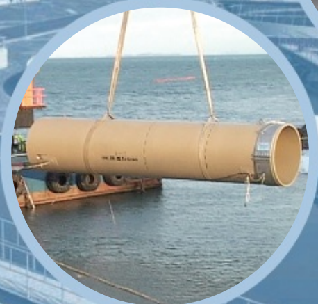
Installation of ocean bed blocks
