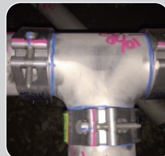
▶ Japan : "T" Repair
