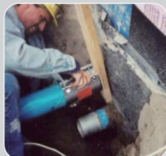
▶ U.S : sewerage repair work
