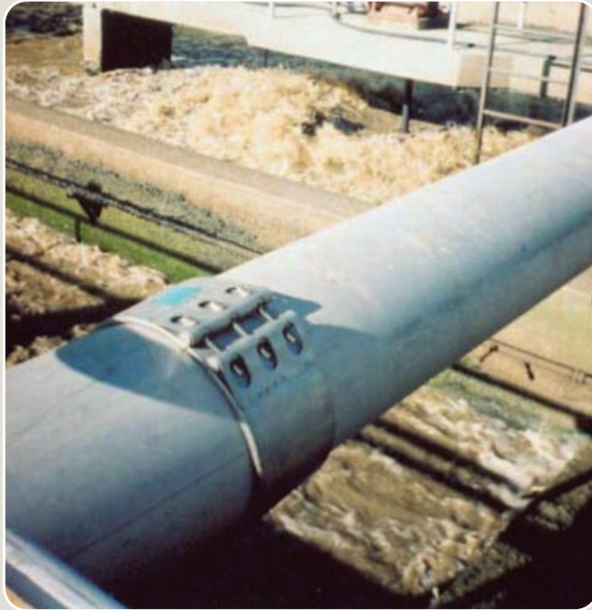
▲ Spain: water purification facilities
