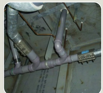
▲ PVC + Steel Pipe Connection
